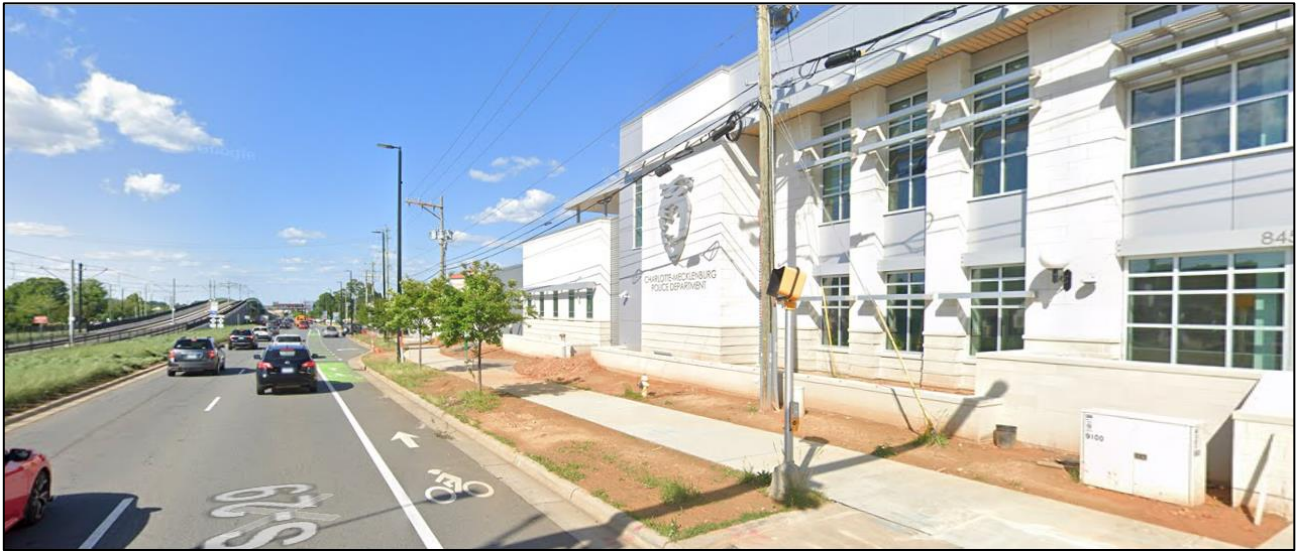
Across and along N. Tryon are institutional, office, residential, and retail uses.
