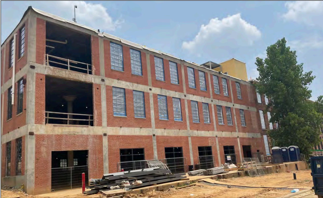
7. West facade of Paper Warehouse, looking E
