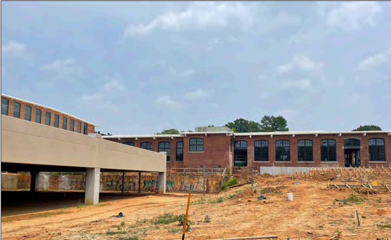
4. West facade of Weave Mill, looking E
