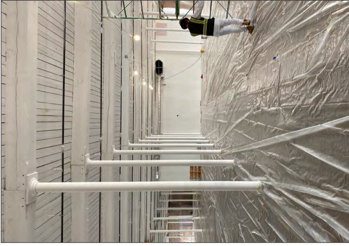
20. Spinning Mill, first floor, looking S toward restroom stack
