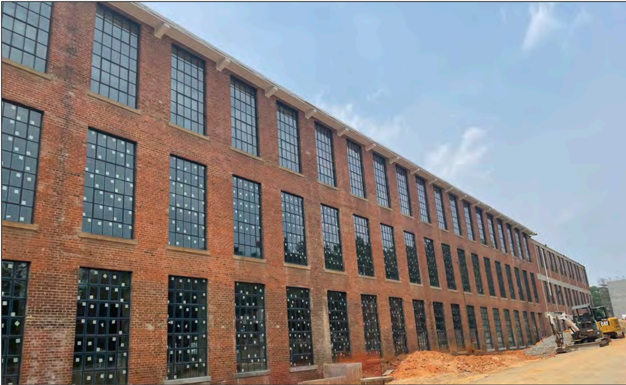
1. Spinning Mill and Paper Warehouse, looking NW
