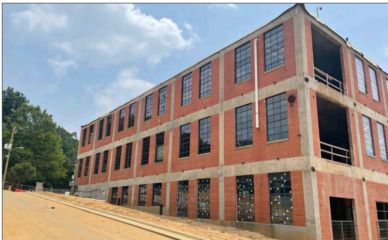
6. North facade of Paper Warehouse, looking SE
