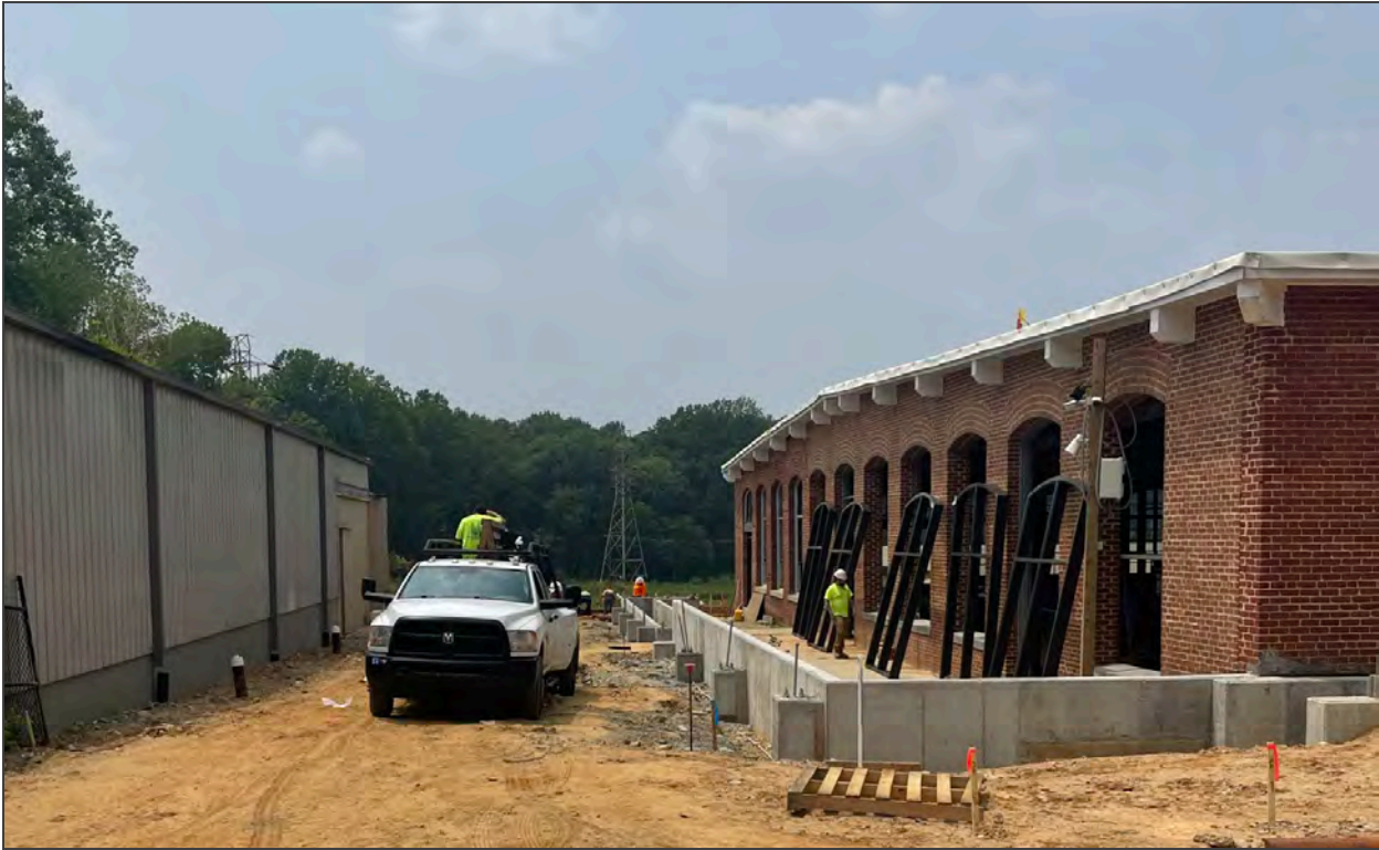
2. South end of Weave Mill, looking W
