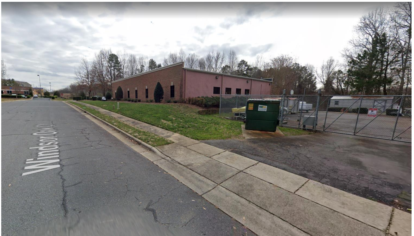
Street view of the site (right side of the picture) looking east of Windsor Oak Ct shows the office space and some outdoor storage buildings for a civil engineering company.
