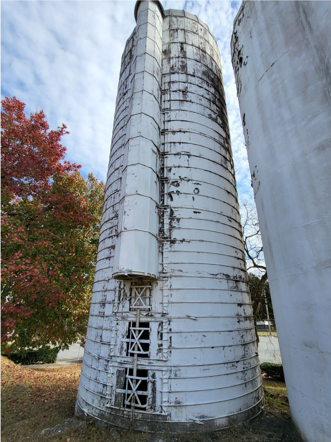
North silo and chute – front/west and south elevation.
