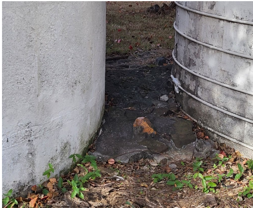
Relative distance between the north (on right) and south (on left) silos.
