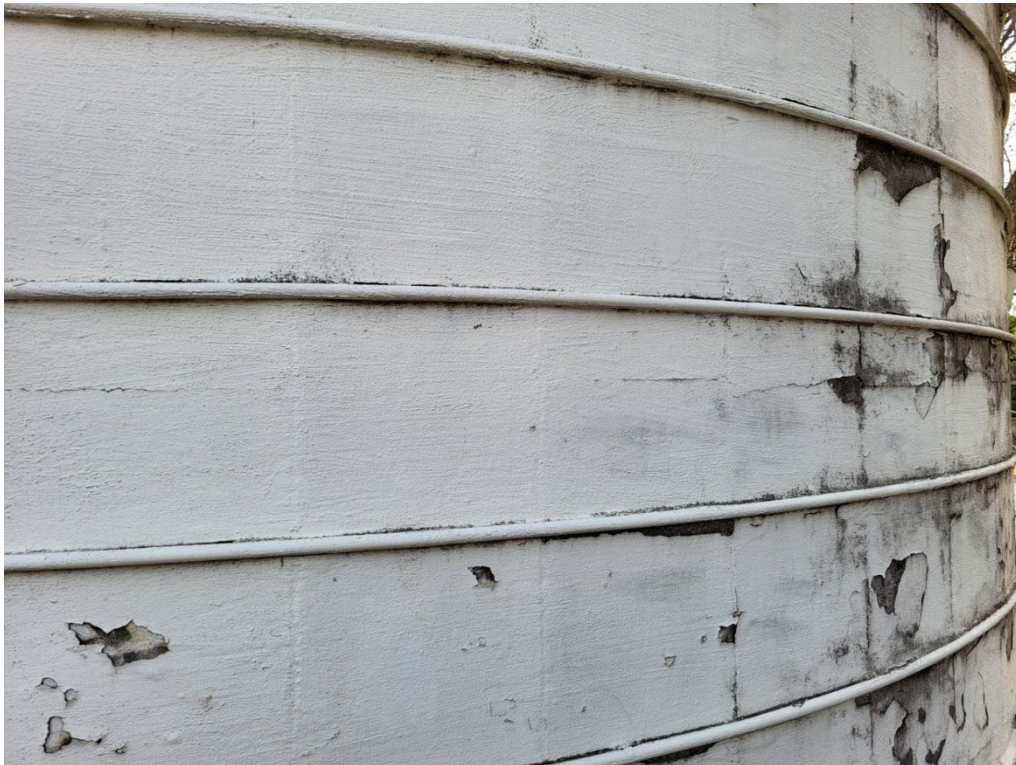
Above: Examples of concrete staves, circa 1919. 56 Below: Detail of south elevation of north silo showing its concrete stave and steel reinforcement hoop construction.
