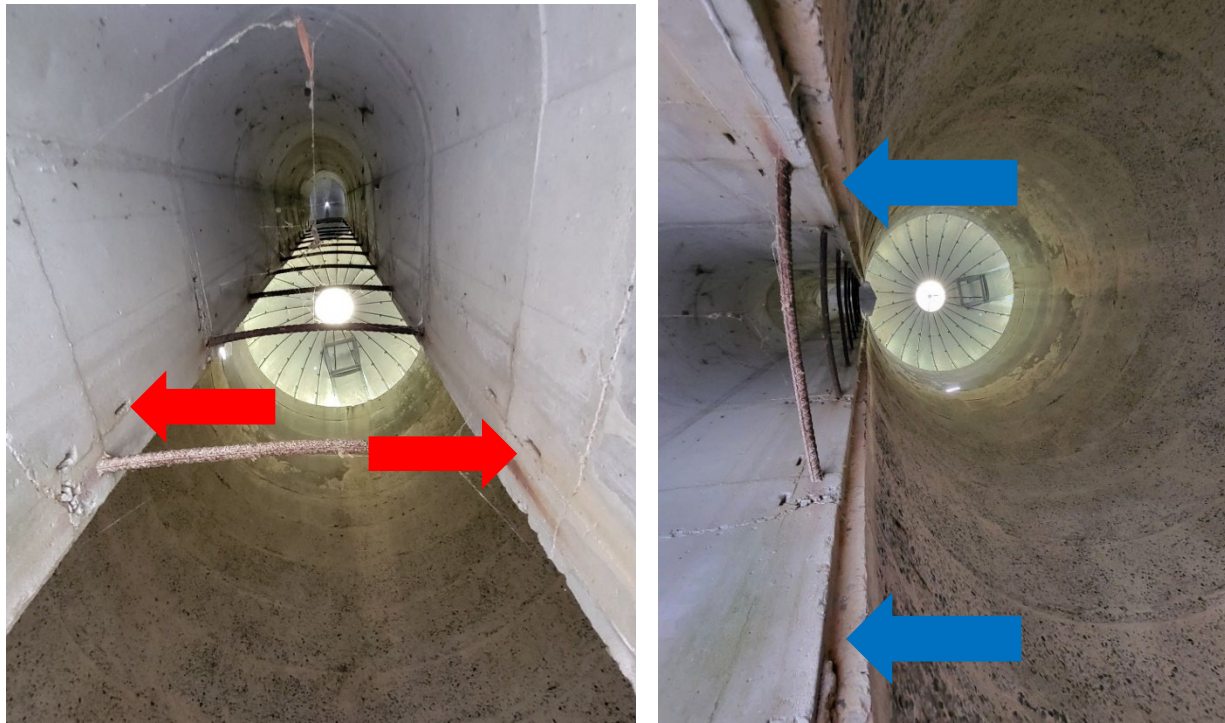
Above: Interior detail of the south silo's chute showing the rebar reinforcing rods and the continuous door extending the full height of the concrete structure. Note the pairs of indentations on either side of the rods (red arrows) and the rabbeted edge of the continuous door's interior (blue arrows), suggesting the earlier presence of some type of mounted barrier to secure the silo's contents. Below: Illustrative example of unloading door component of continuous door construction.
