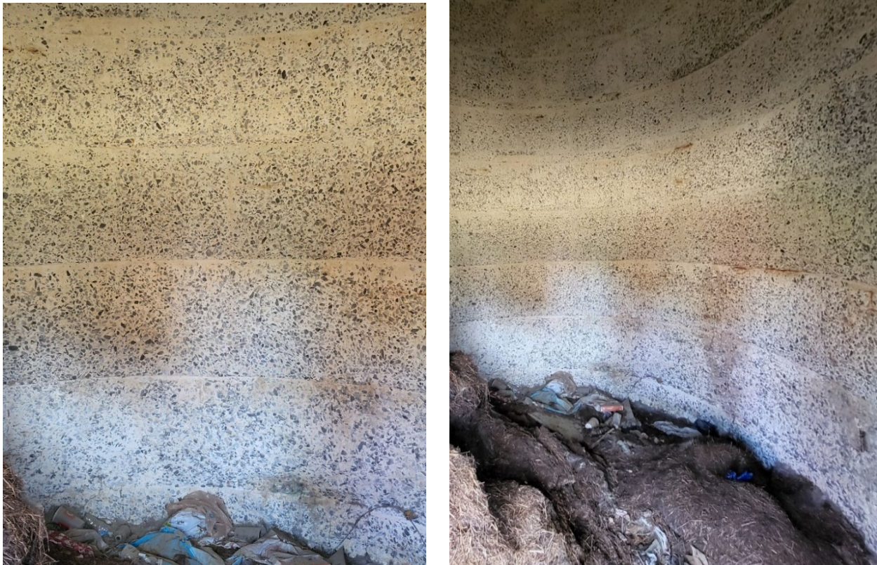
Interior walls of south silo.
