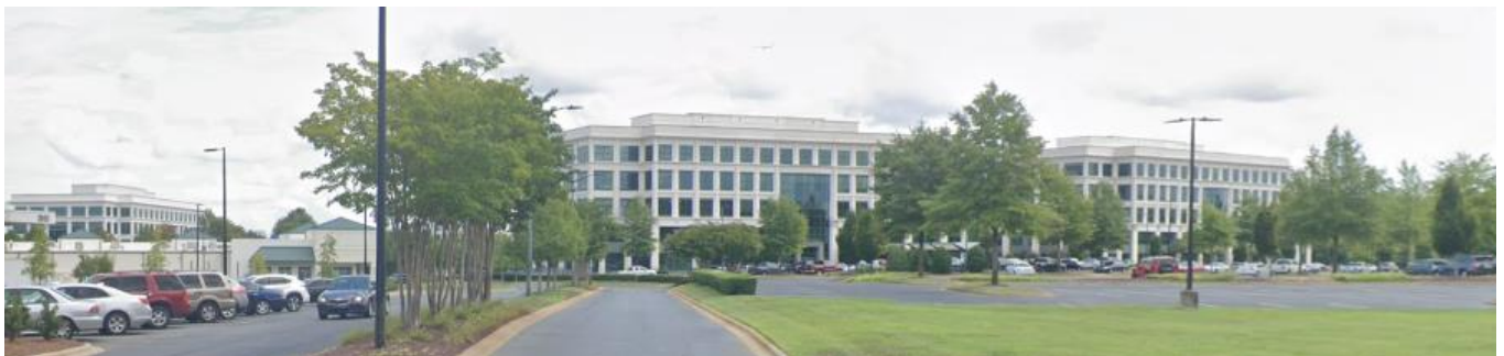
Street view of properties to the north of the site along Arco Corporate Circle developed with retail and office uses.
