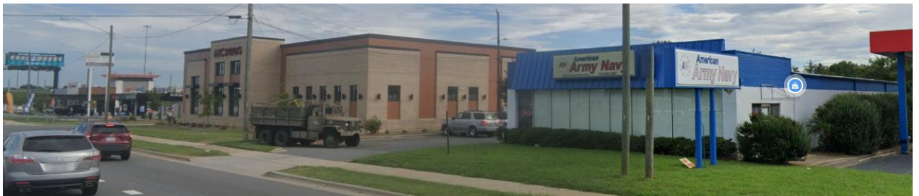
East of the site are commercial uses along Independence Bv.
