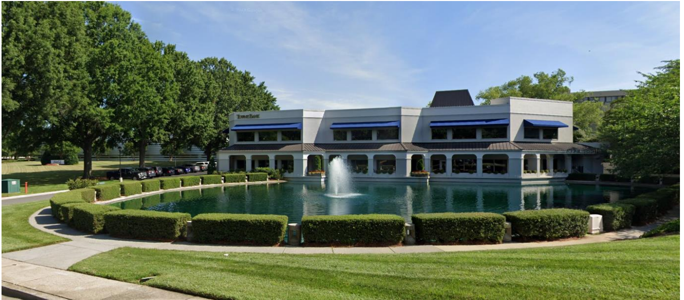
The site is currently occupied by an office building.
