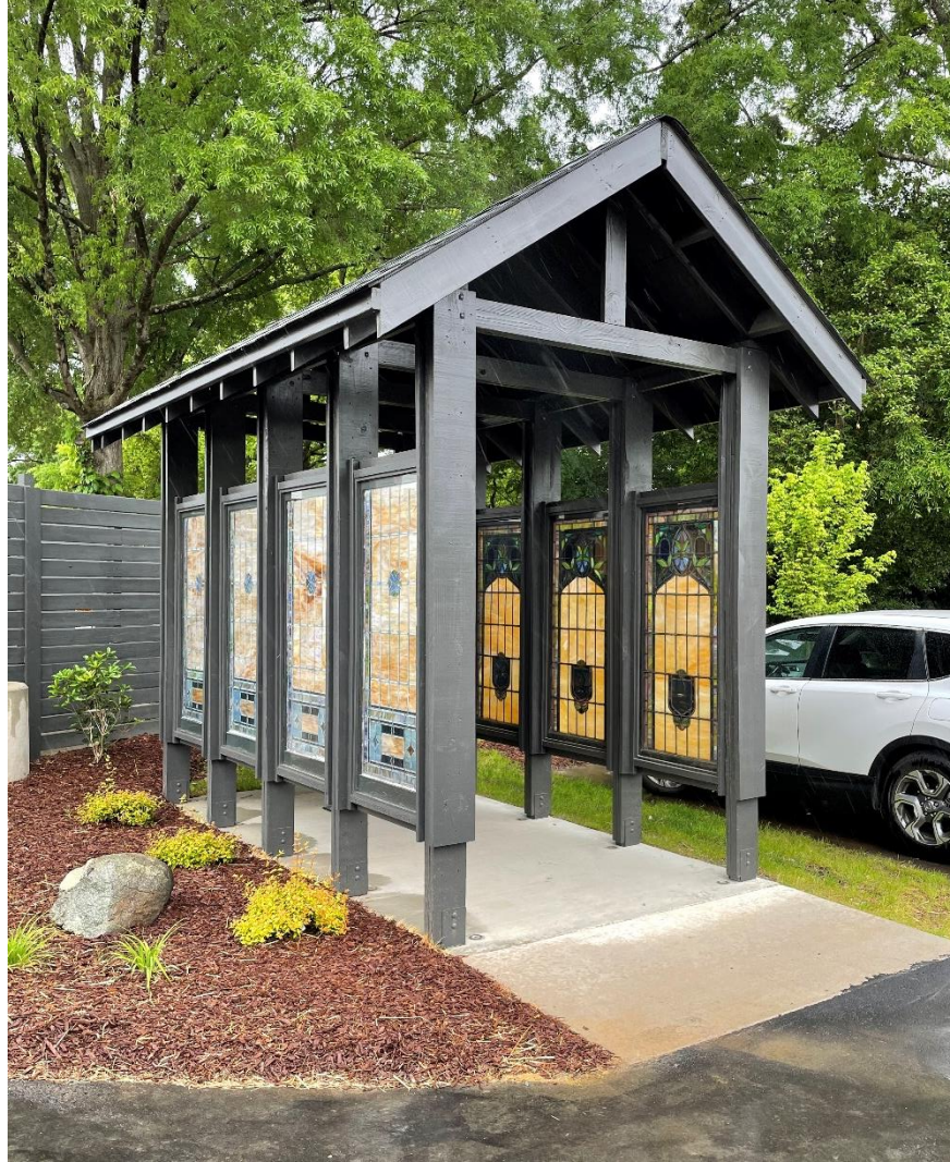
Figure 19 The mail pavilion incorporates stained glass panels from the former church, 2021.
