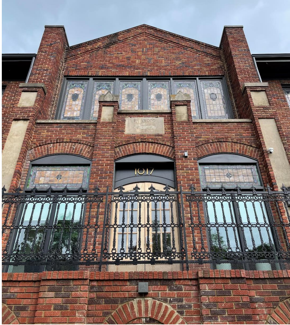
Figure 12 Center bay of the south elevation.
