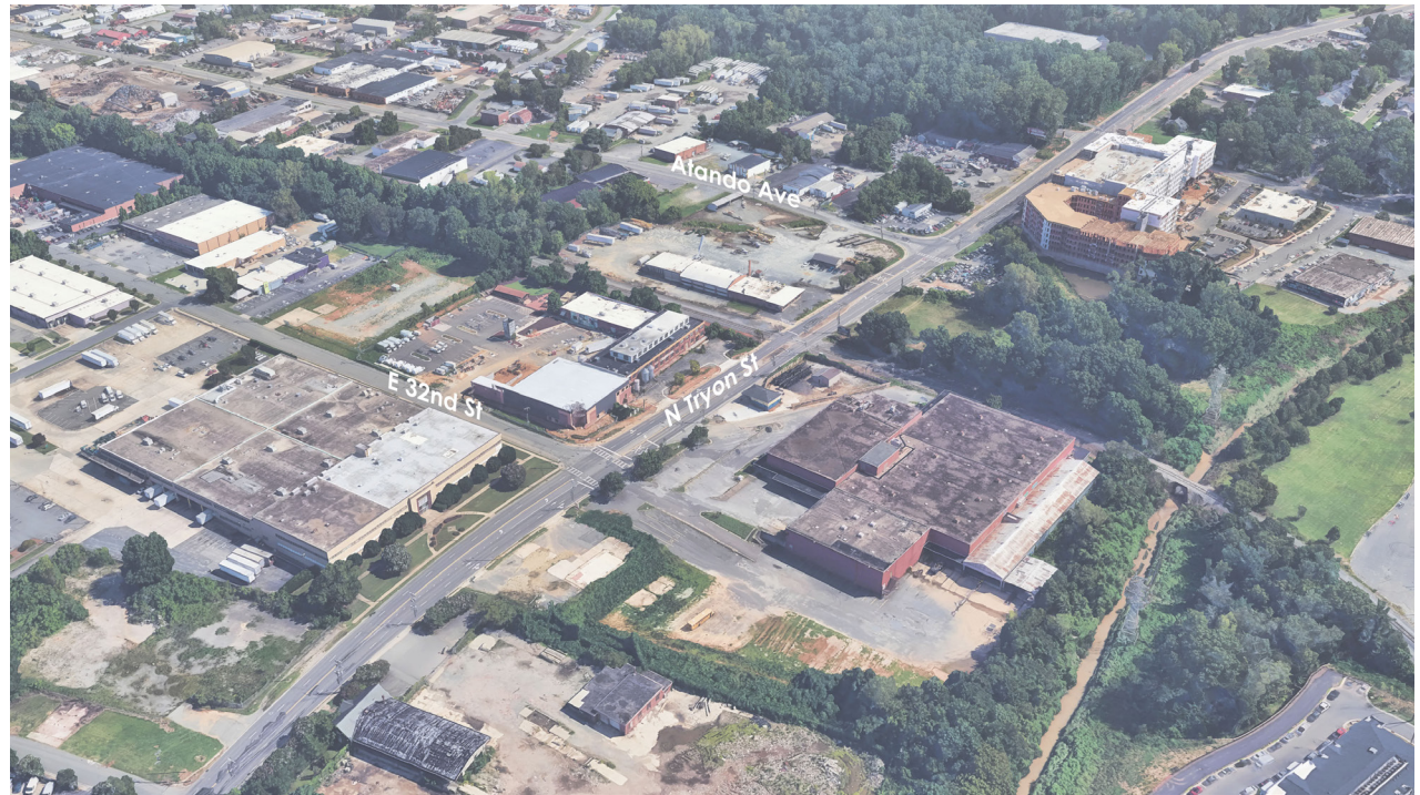
FIGURE 11: AERIAL OF EXISTING CONDITIONS
