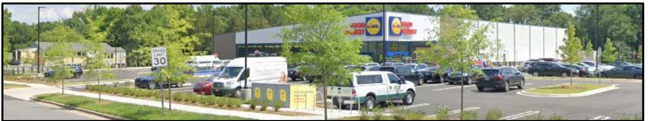
South of the site, across Carmel Commons Boulevard is a grocery store, personal service and day care use.
