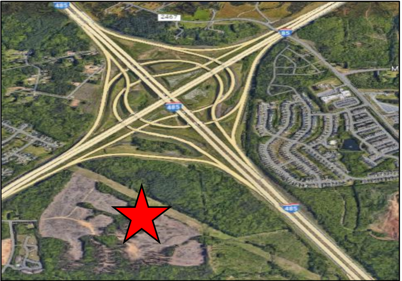
The property to the north of the site are the Interstate 485 and Interstate 85 interchanges.
