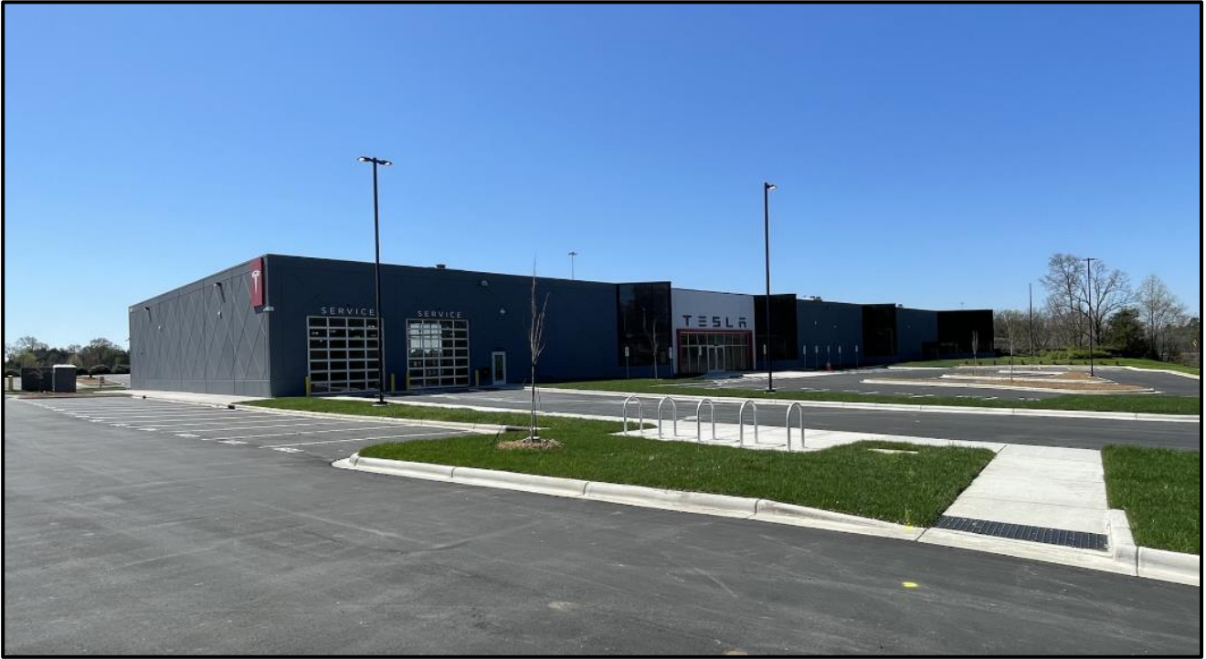
The property to the south along Twin Lakes Parkway is developed with a Tesla auto dealership.
