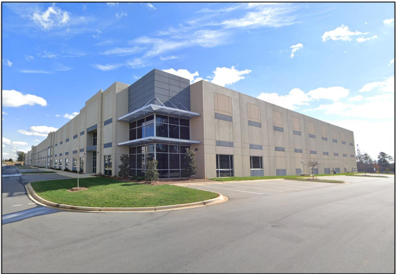
South of the site is an industrial use building.
