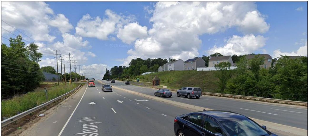
West along N. Tryon Street are single family residential neighborhoods, commercial uses, and vacant land.
