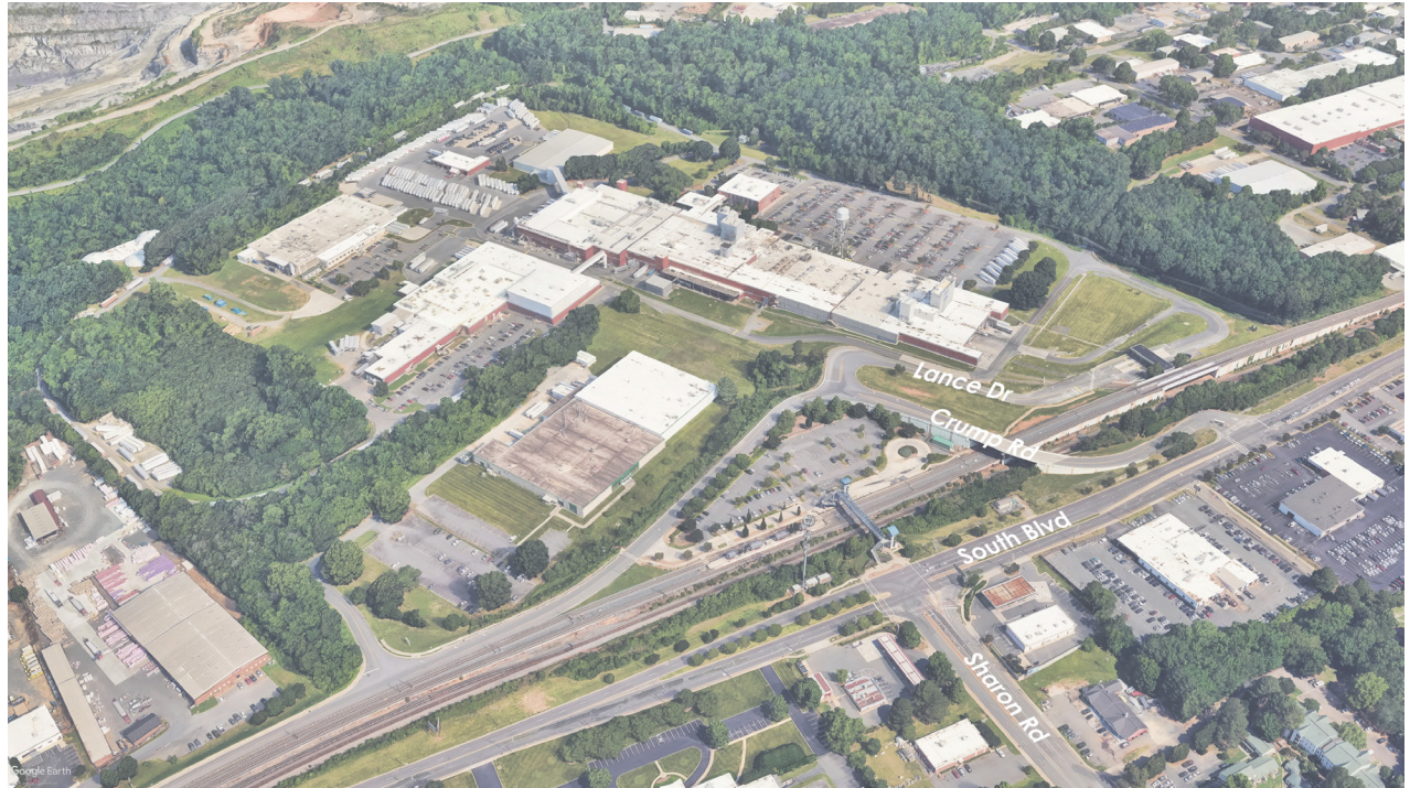
FIGURE 11: AERIAL OF EXISTING CONDITIONS
