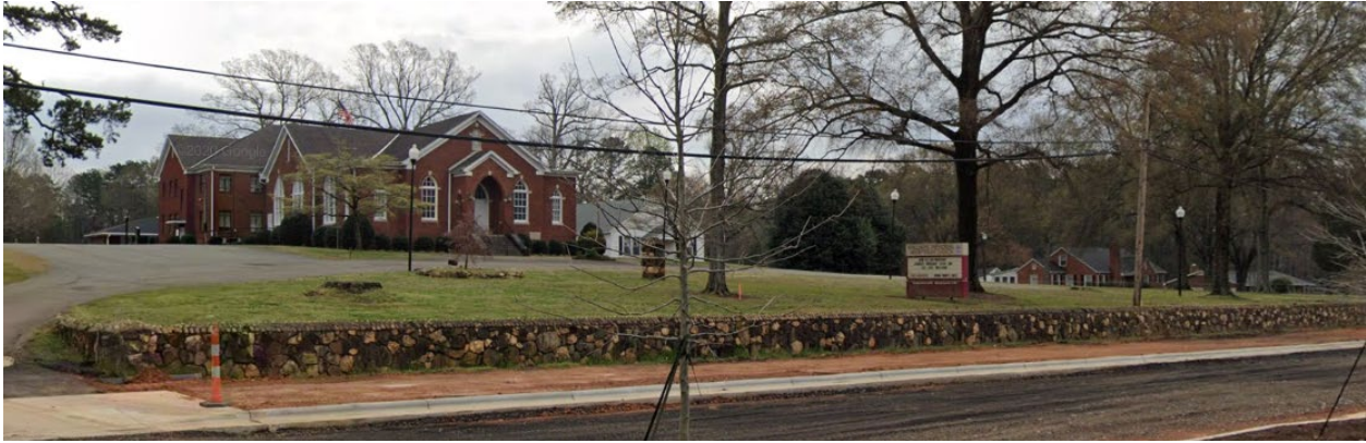
West face of Williams Memorial Presbyterian Church Wall
