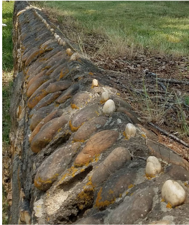
Detail of Domed Cap of Williams Memorial Wall
