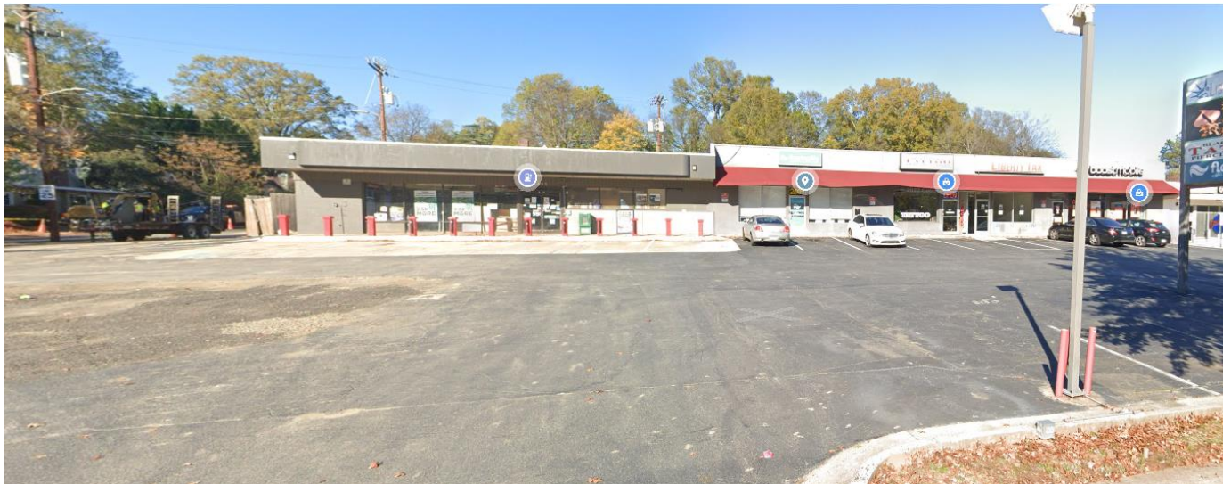
The site is developed with a multi-commercial tenant building (above) and a single family home (below).
