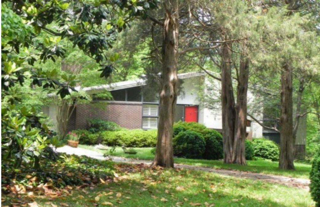
Winecoff House, 6631 Williams Road
