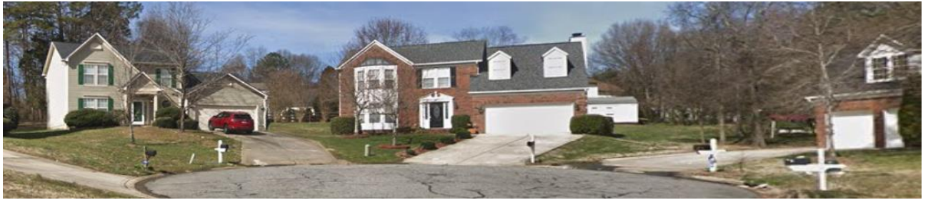
The properties to the west of the site are developed with single family residential uses.
