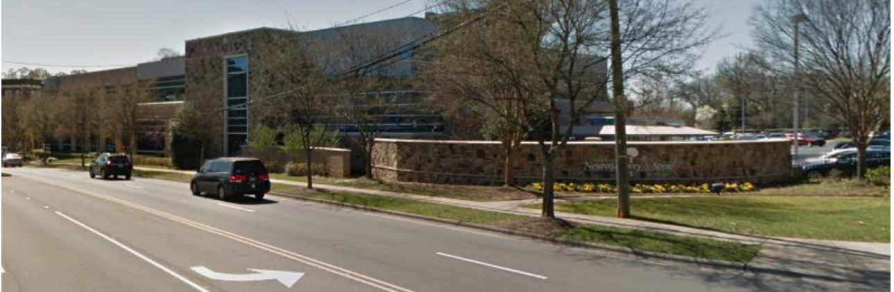
The property across E. 3 rd Street is developed with a medical office.
