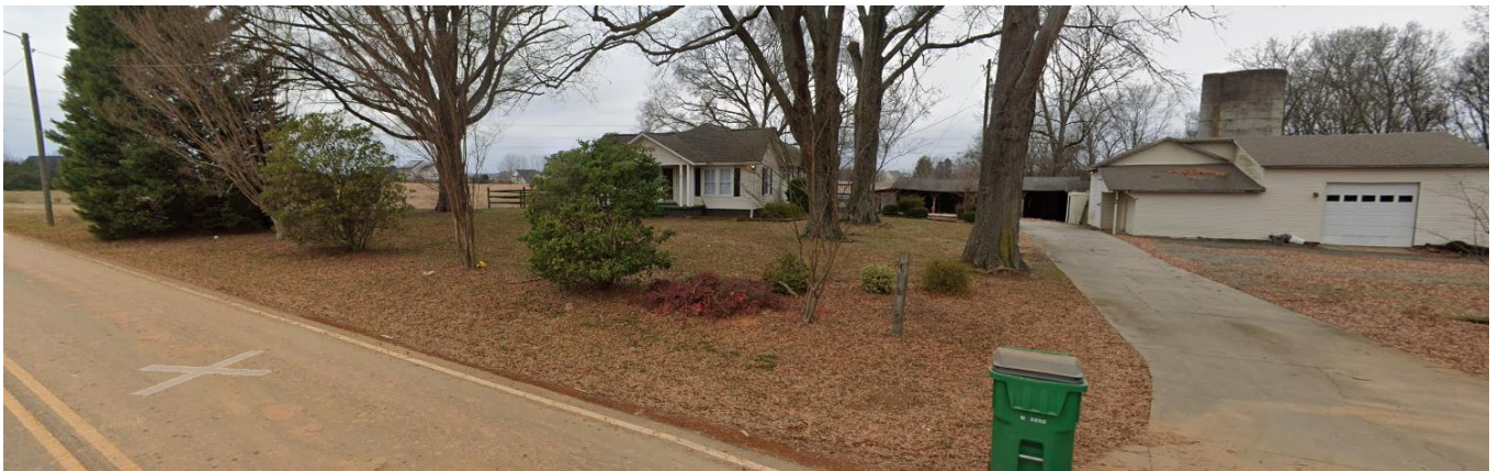
The rezoning site is developed with residential structures, a pond, and vacant land, and is surrounded by single family detached and multi-family residential communities.
