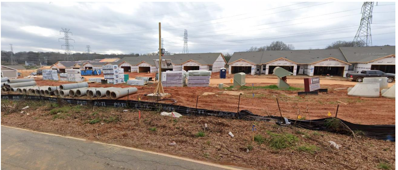
South is a multi-family residential community under construction.
