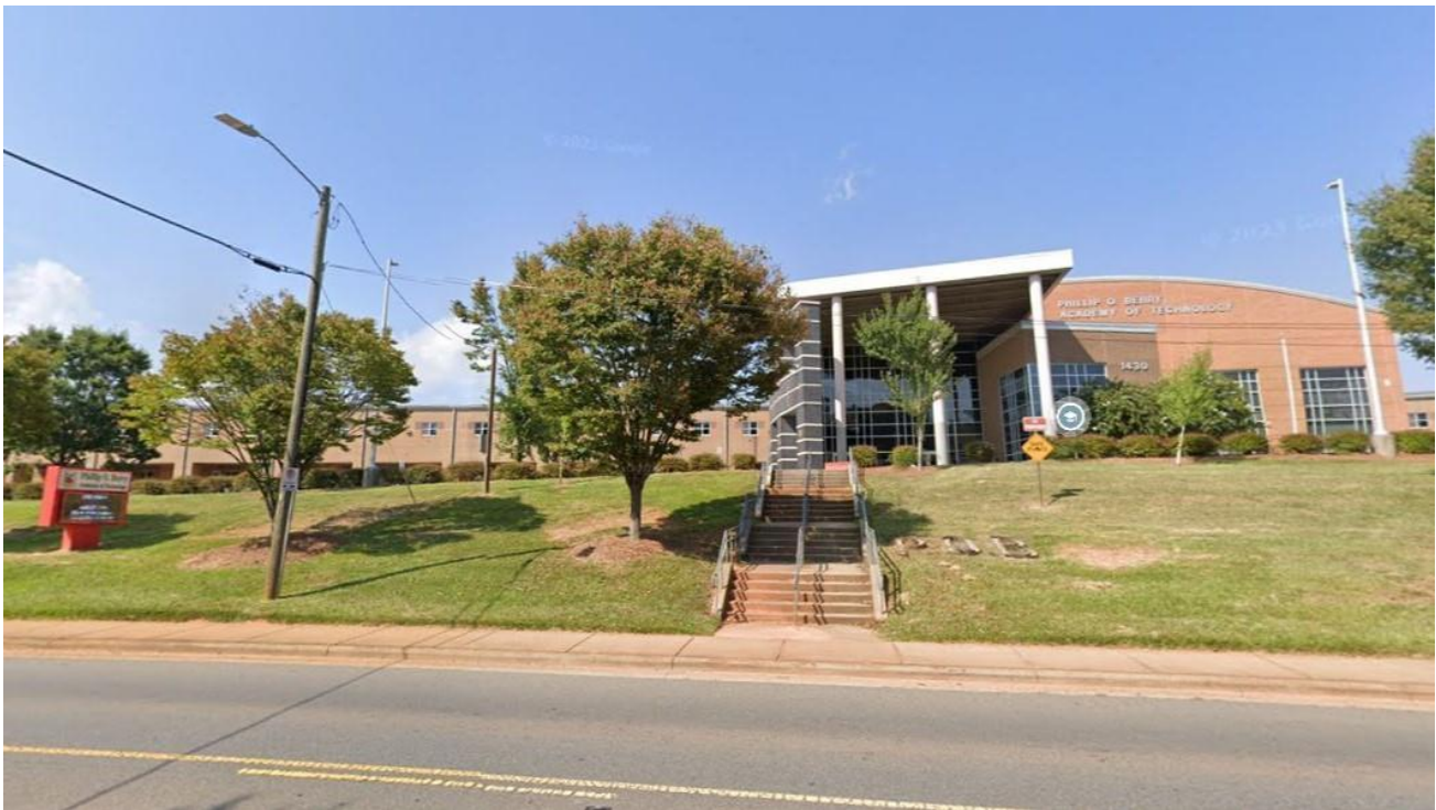
View of the Philip O. Berry Academy of Technology located on Allegheny Street east of the site. There are three schools located within a 1/2-mile walking distance of the site including Harding University High School and Ashley Park Elementary School.
