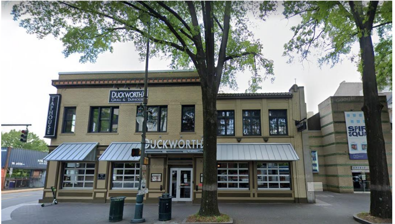
The properties to the north of the site are developed with a restaurant and a performing arts theater.
