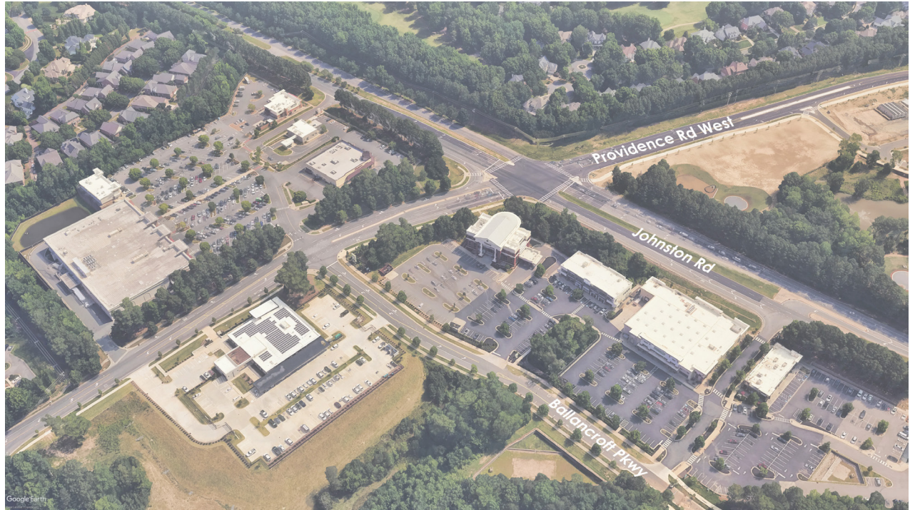
FIGURE 11: AERIAL OF EXISTING CONDITIONS
