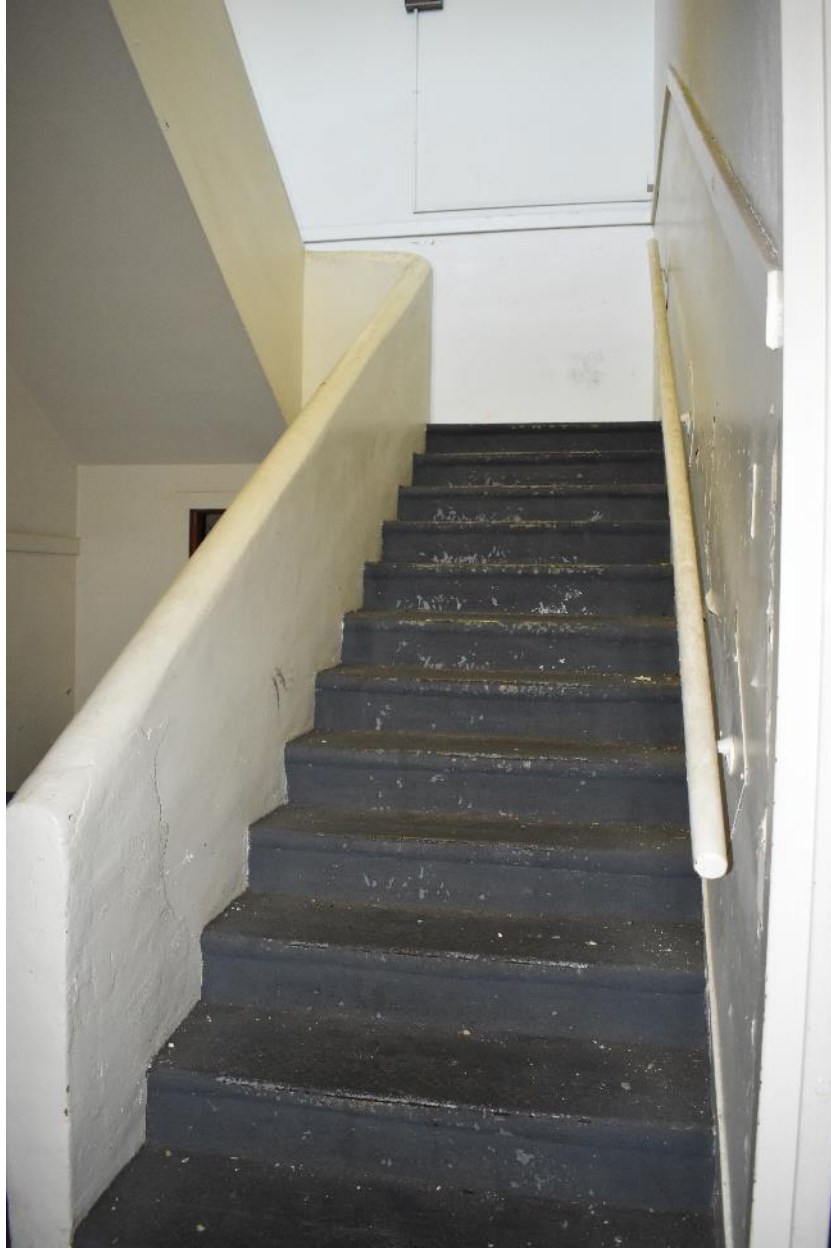
East stairwell, located in the original 1925 building.
