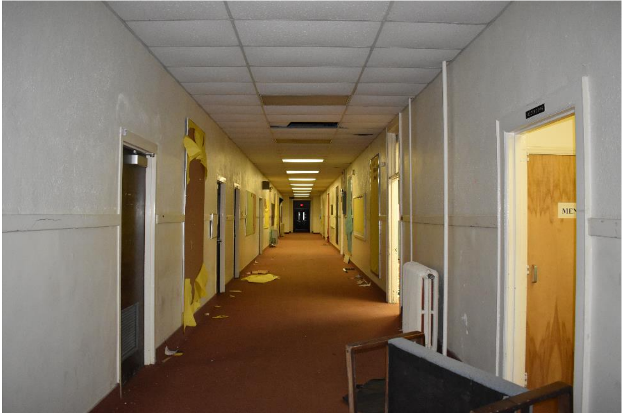
First floor hallway of the original 1925 building looking east to west.
