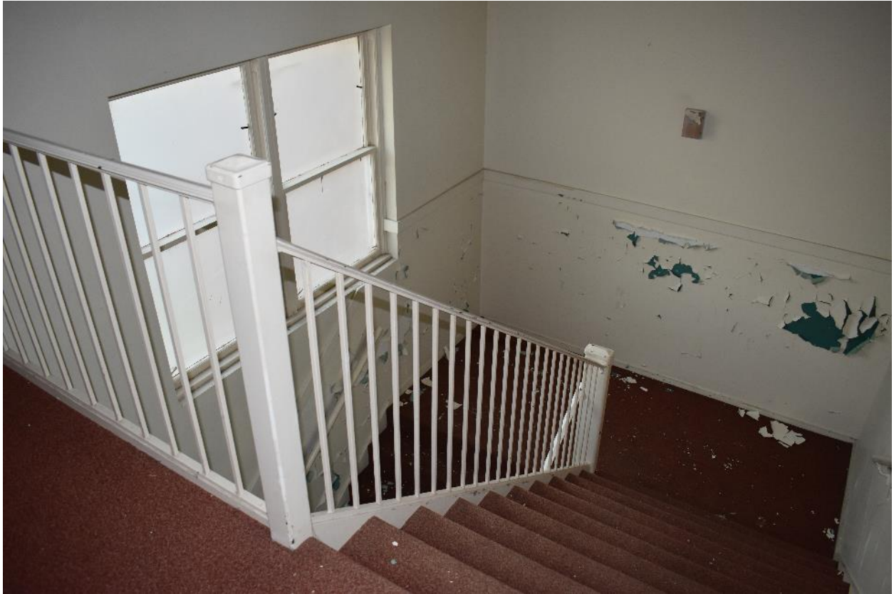
West stairwell looking northeast, located in stair/bathroom tower of the 1948 addition
