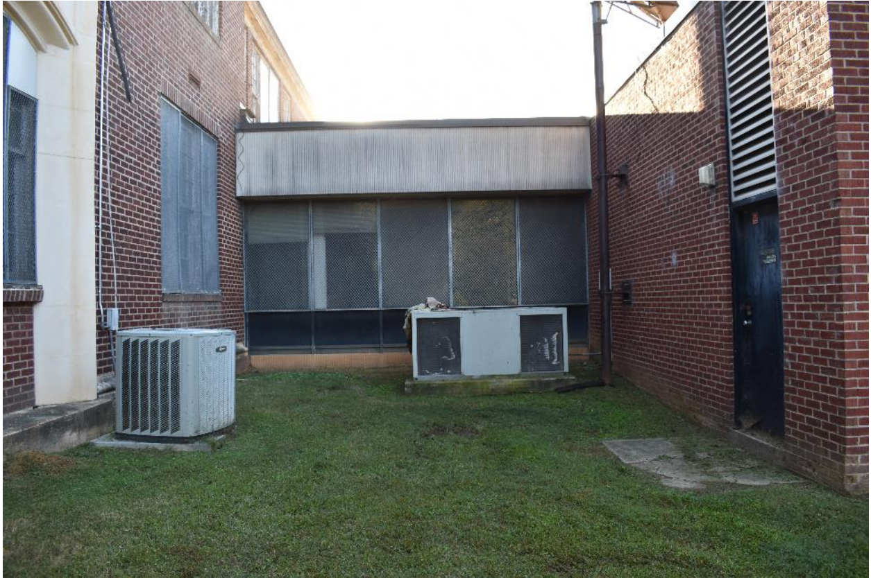
West elevation of the 1970 library/administrative addition.
