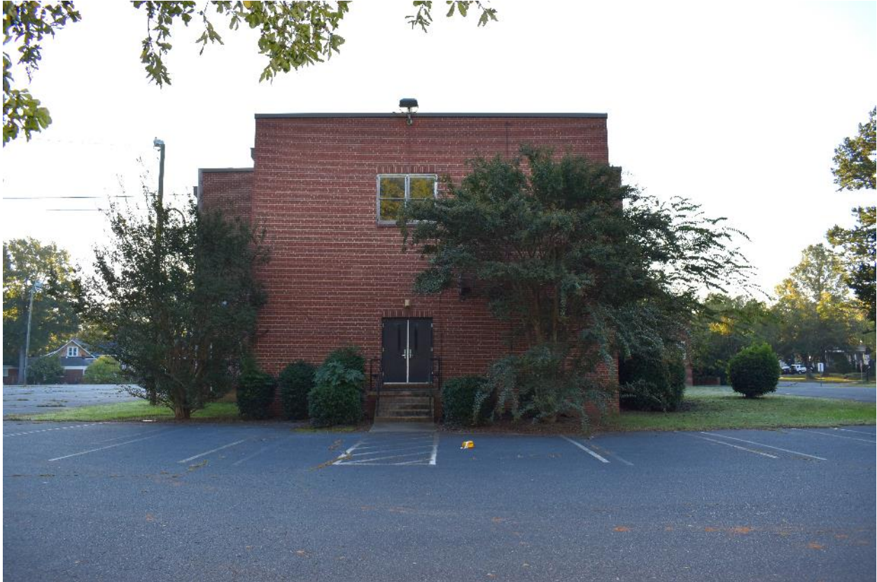
West elevation of the 1948 stair/bathroom wing.
