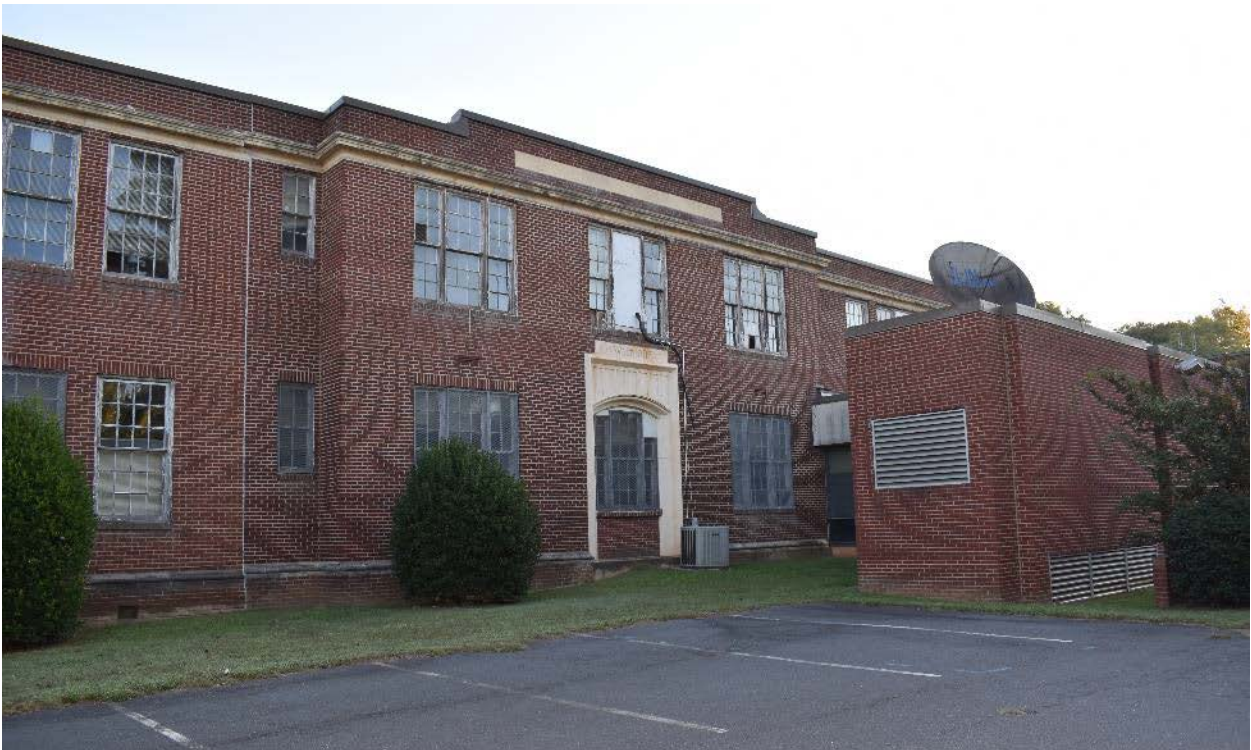
South elevation of 1925 original building and 1948 classroom addition with 1970 library/administrative addition visible.
