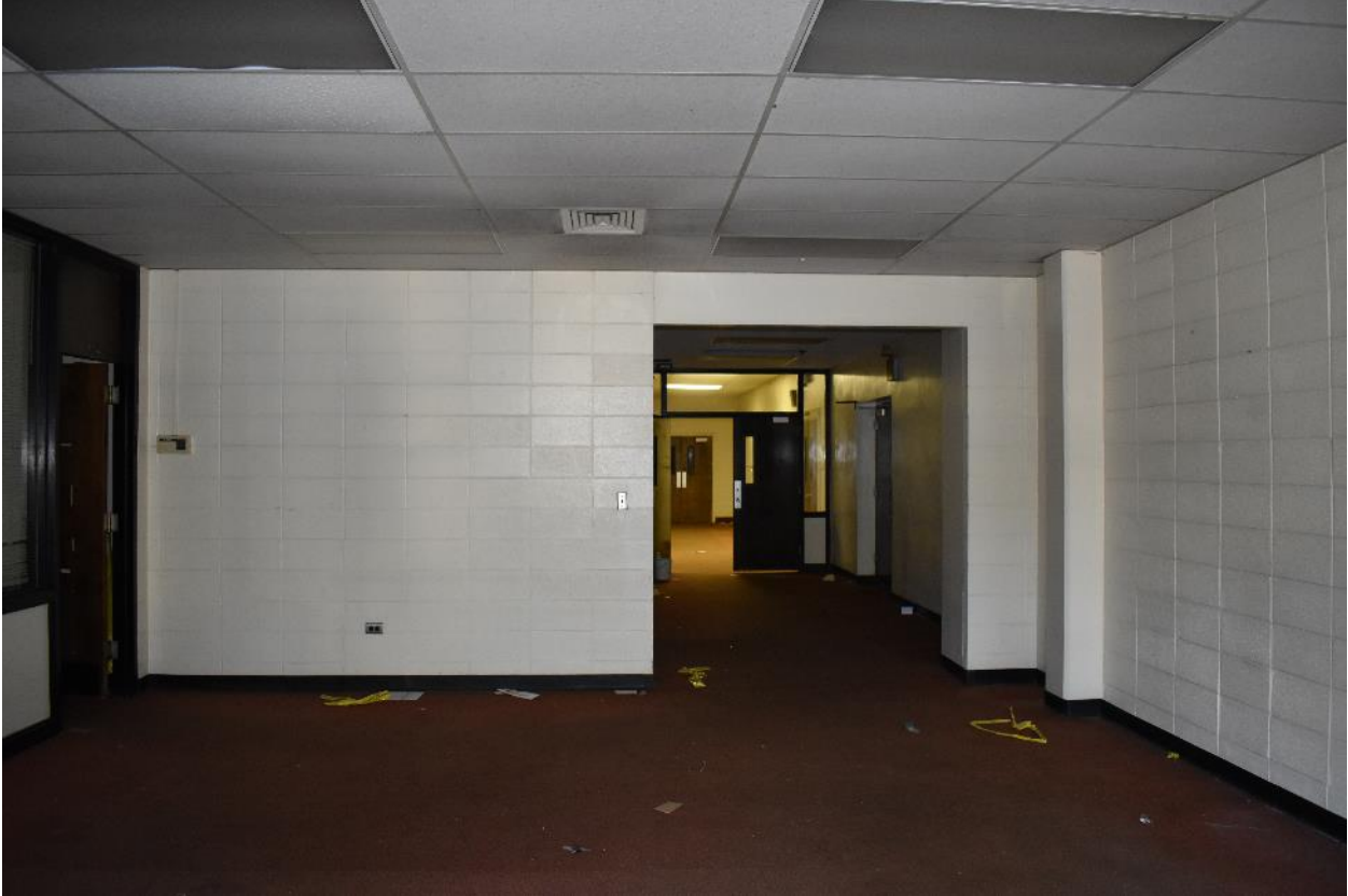
Entrance foyer and administrative section of 1970 library/administrative addition looking north.
