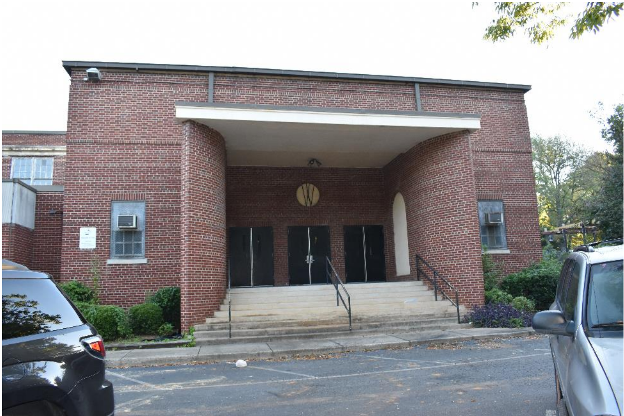
South elevation of the 1948 auditorium.
