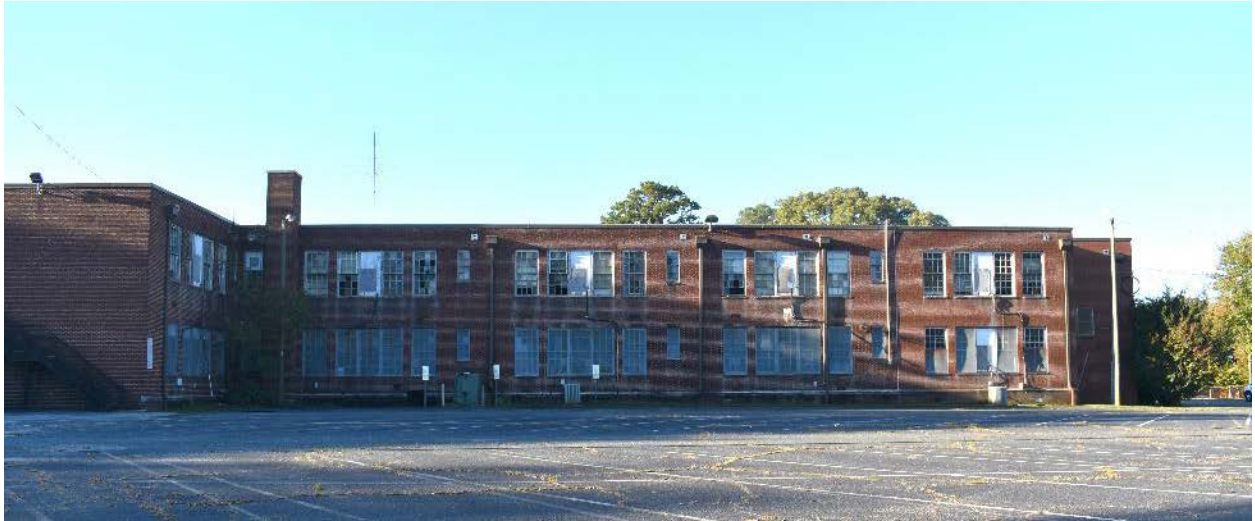
North elevation of the 1925 original building and 1948 classroom addition.
