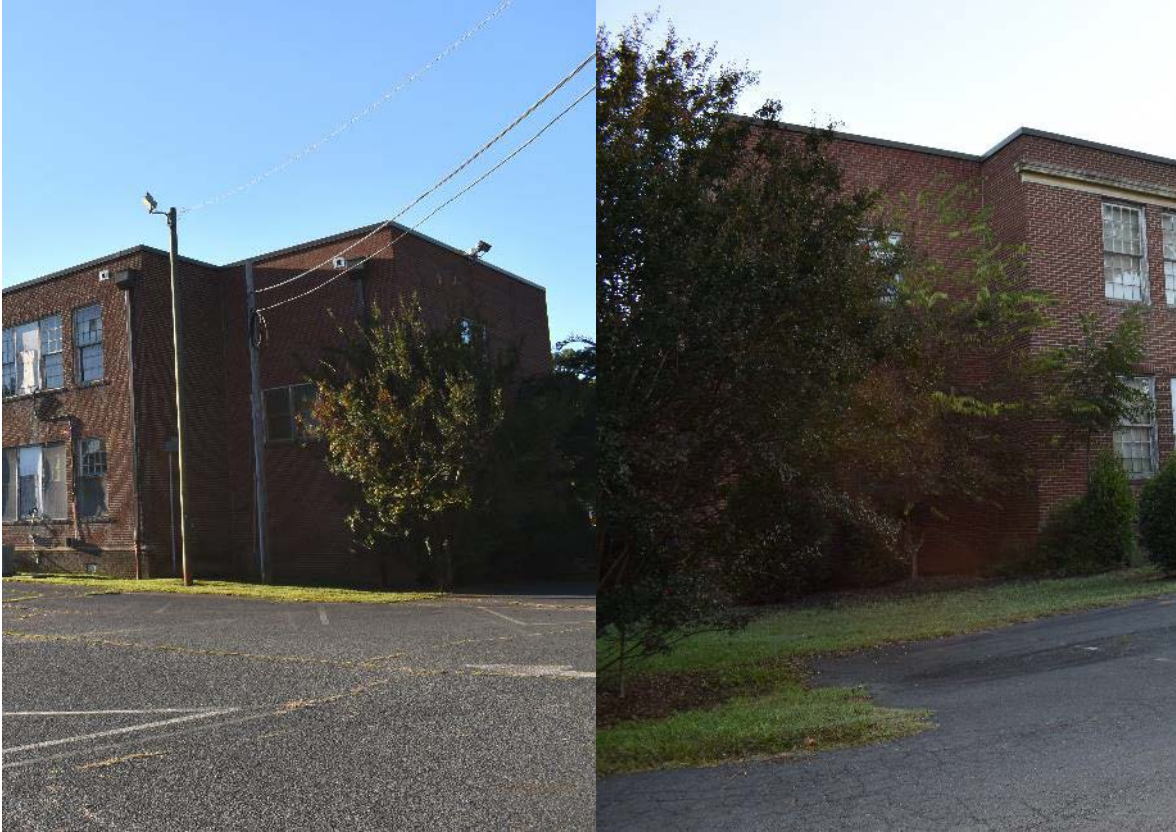
North (left) and south (right) elevations of the 1948 stair/bathroom wing.
