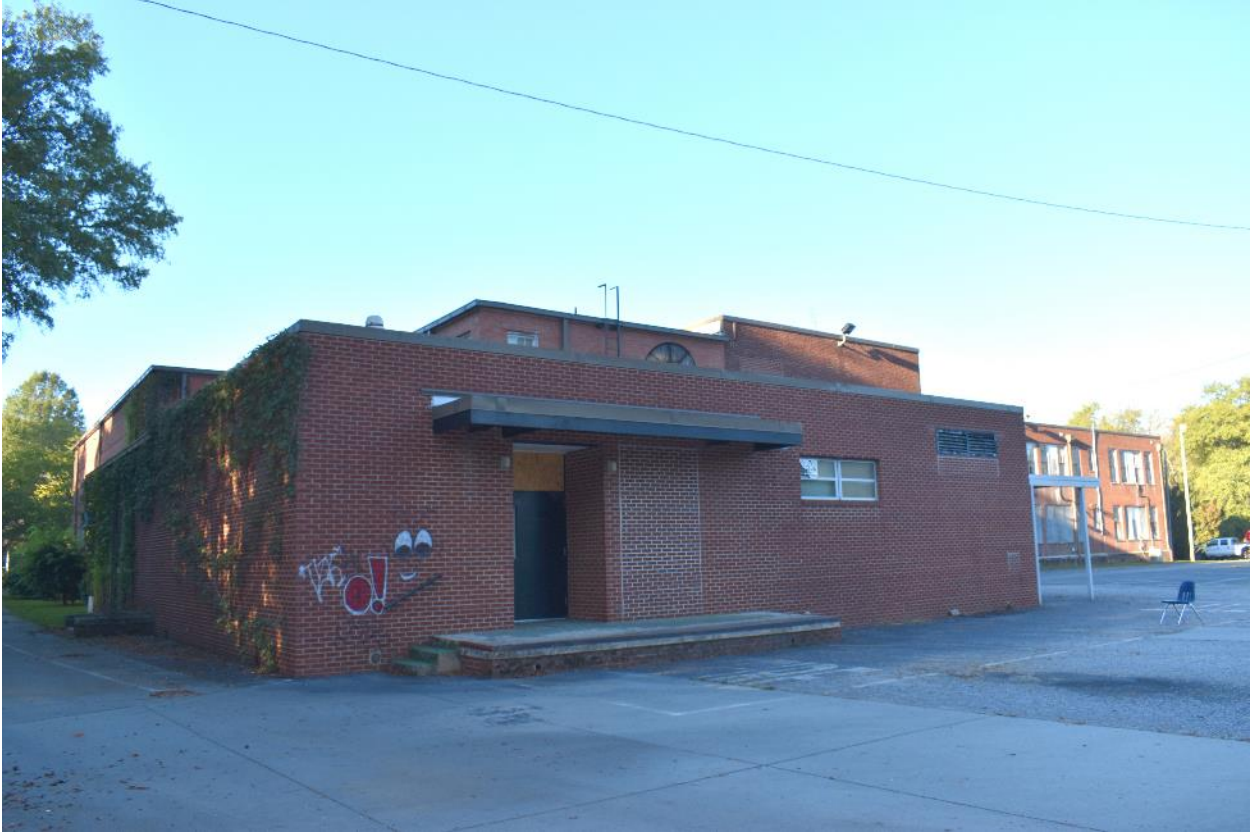
East and north elevation of the cafeteria addition.
