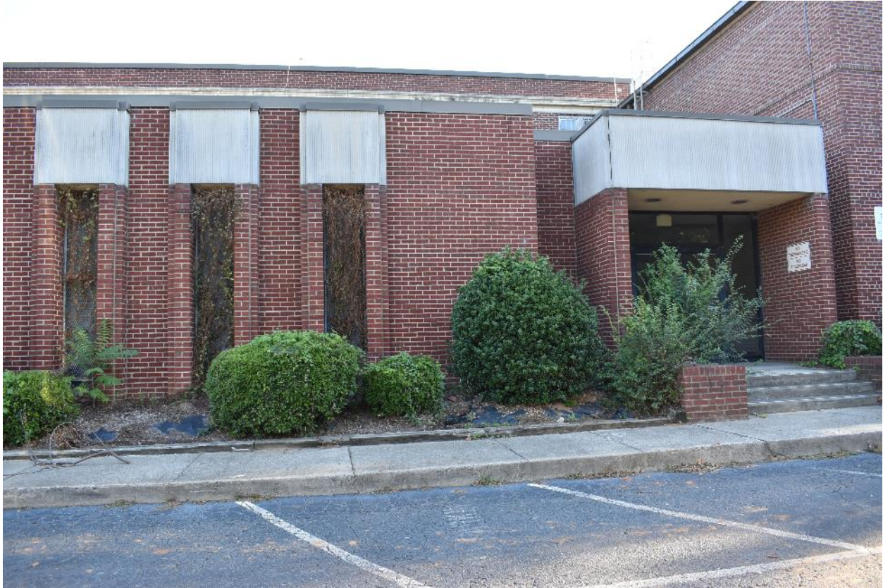
South elevation of the 1970 library/administrative addition.
