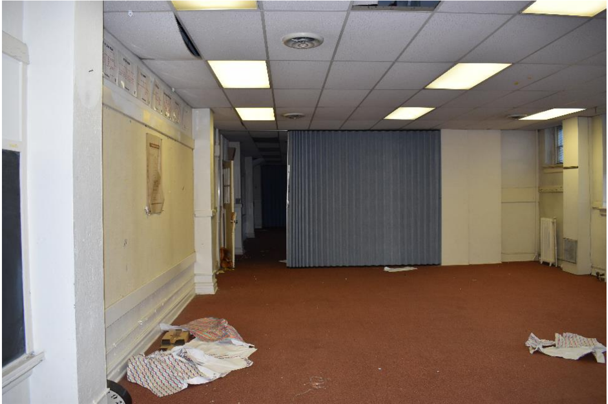
First floor cluster classroom (1970 alteration) looking west.
