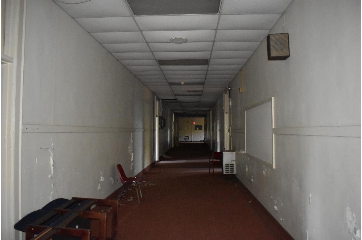
Second floor hallway, looking east from the 1948 classroom addition.
