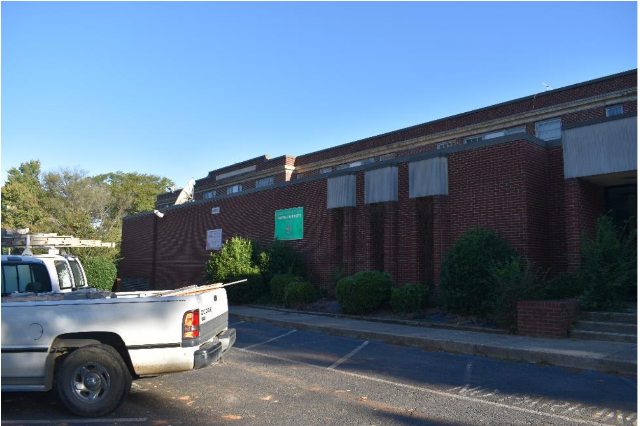
South elevation of the 1970 library/administrative addition.
