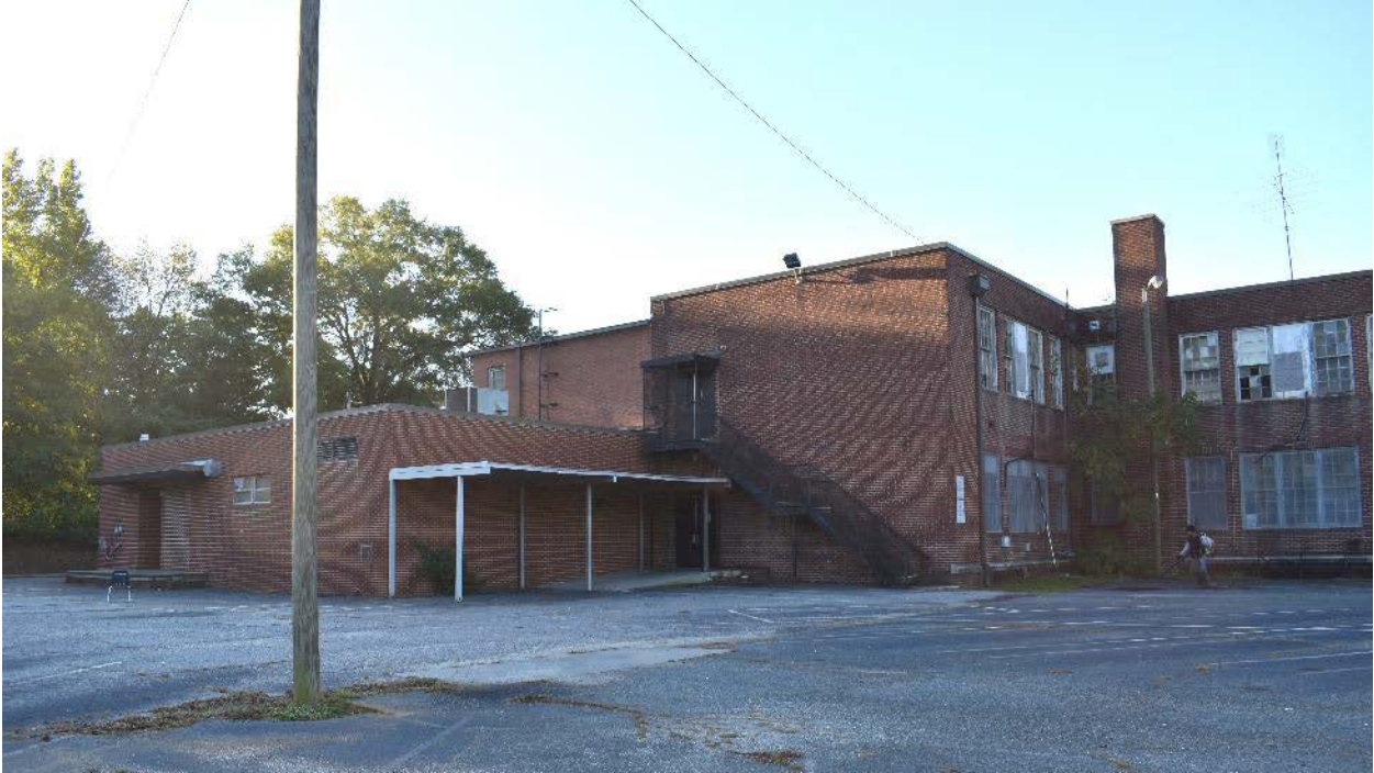
North elevation of the cafeteria addition and the north wing of the original 1925 building.
