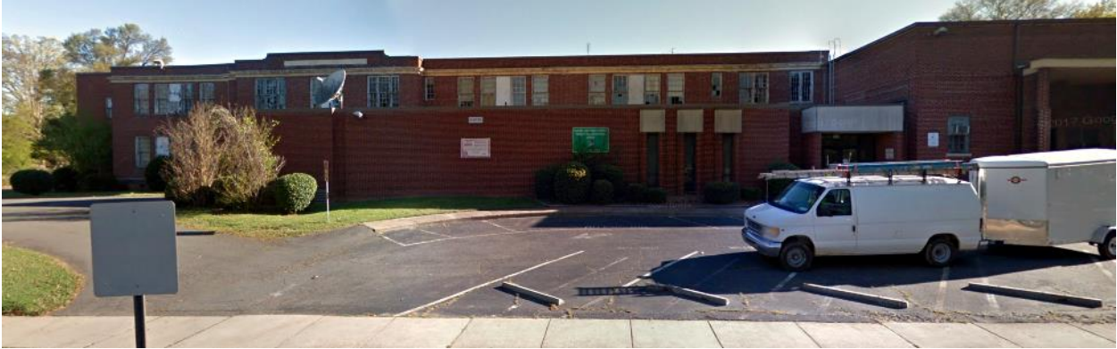
South elevation showing 1925 original building, 1948 classroom addition, 1970 library/administrative addition, and 1948 auditorium.
