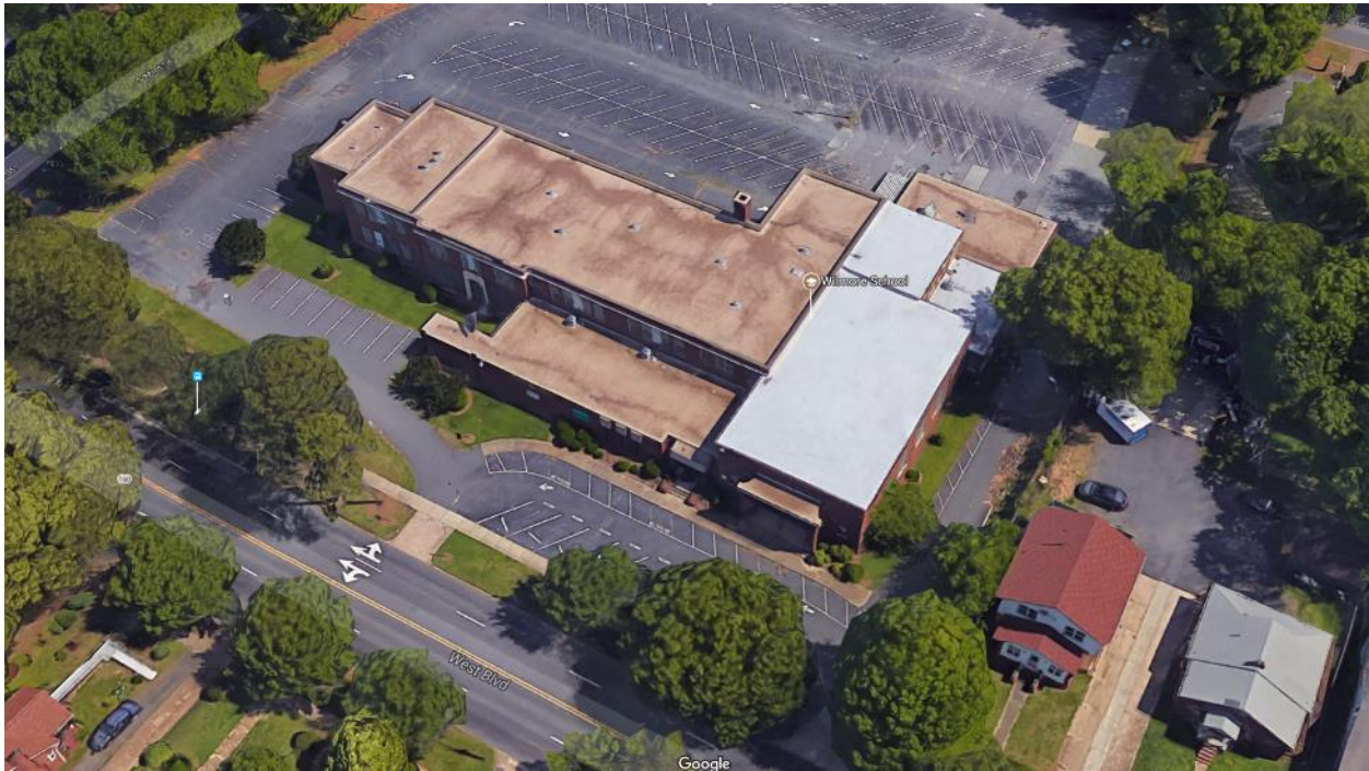
Aerial view of Wilmore Elementary School looking north.
