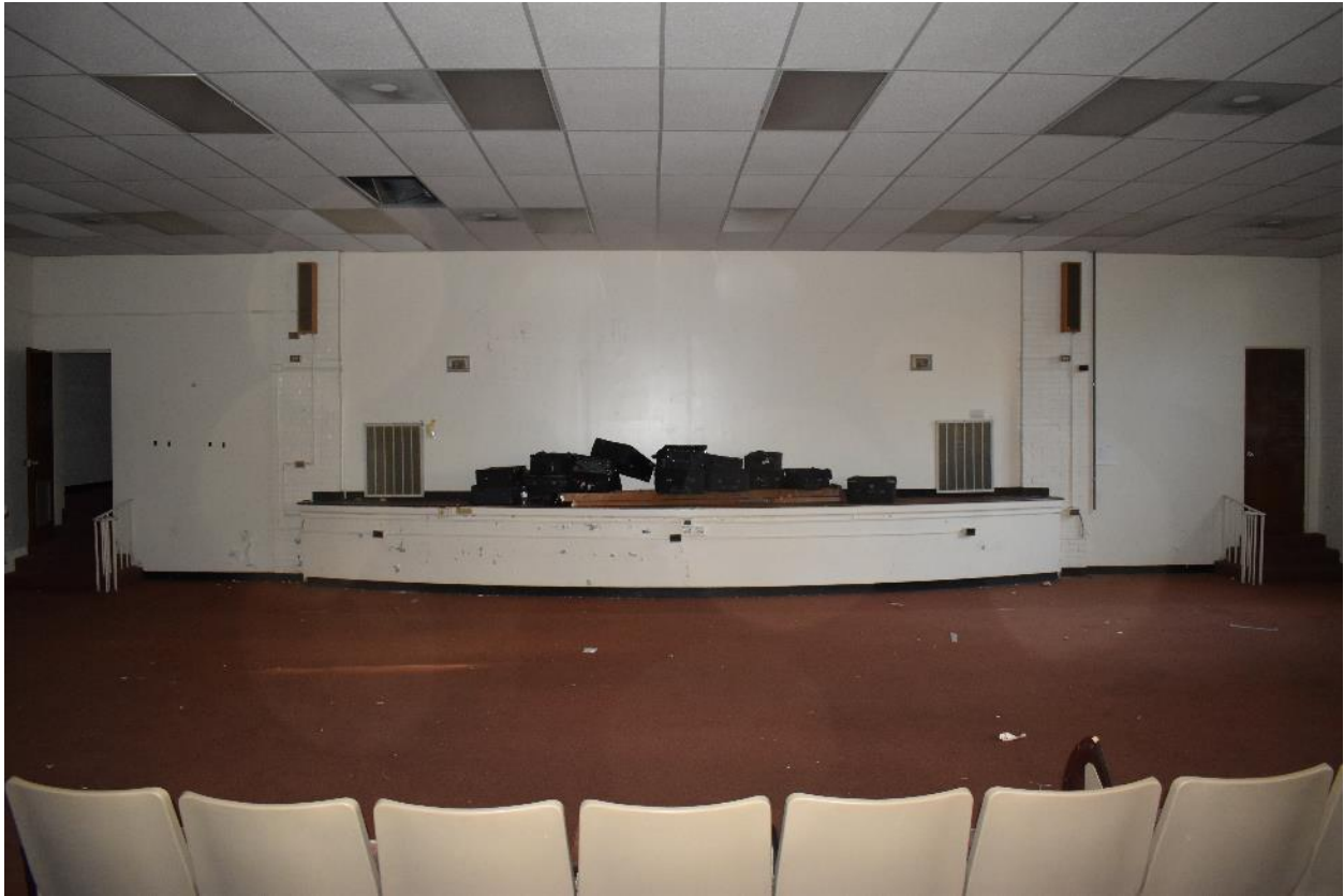
1948 auditorium looking north.
