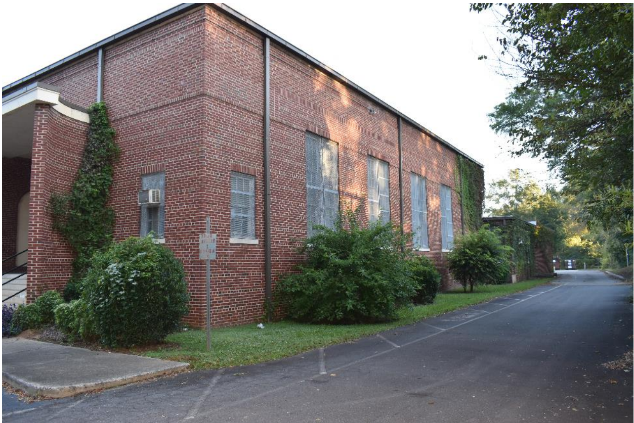
East elevation of the 1948 auditorium and 1948 and 1970 cafeteria addition.
