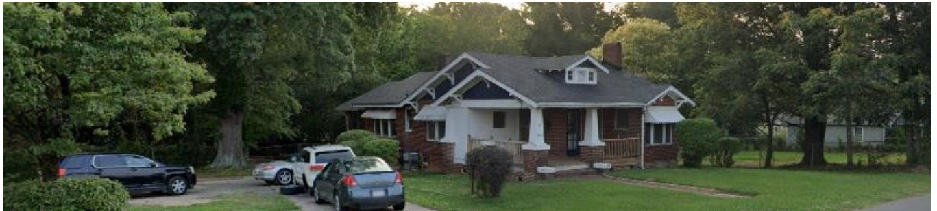
Street view of the site from Westery Hills Drive. The site is currently occupied by a single family dwellings.
