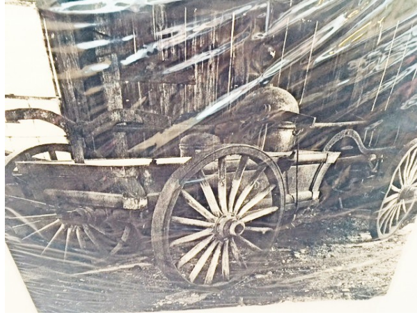
Neptune Pumper Showing Damage From 1910 Fire.
