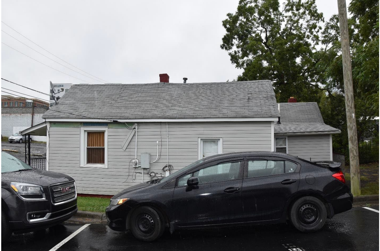
Figure 17 The right elevation looking east.
