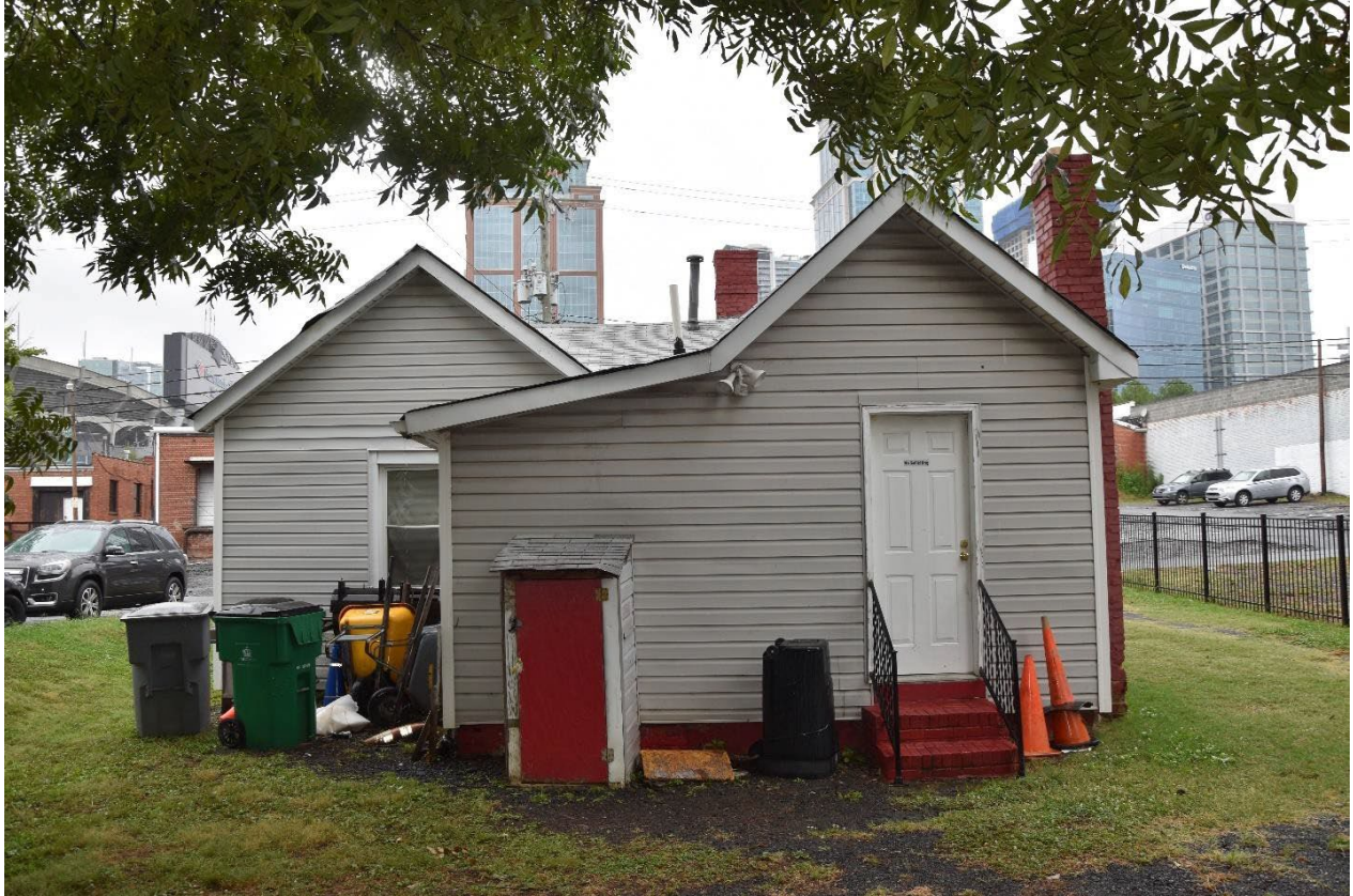
Figure 18 The rear elevation looking north.
