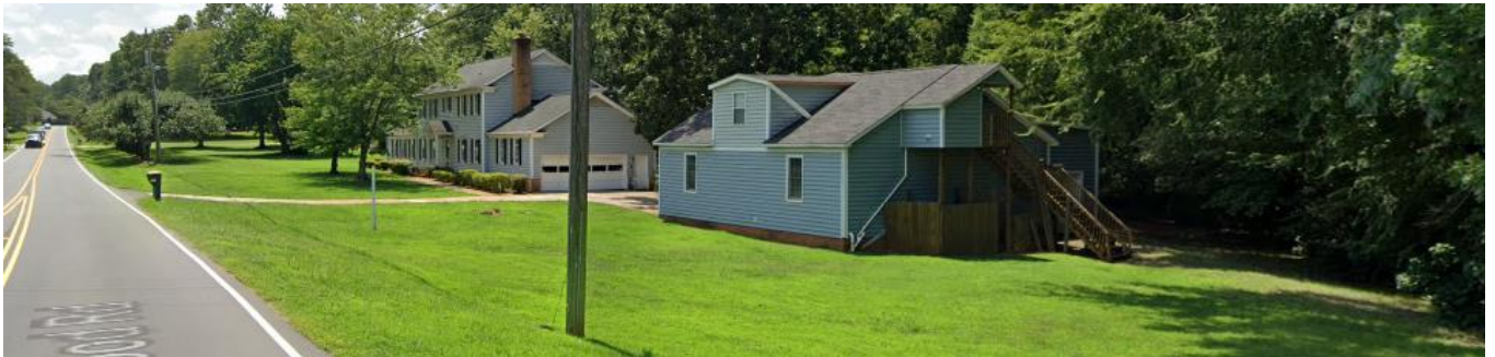
Streetview of single family detached residential uses to the south of the site along Youngblood Road.
