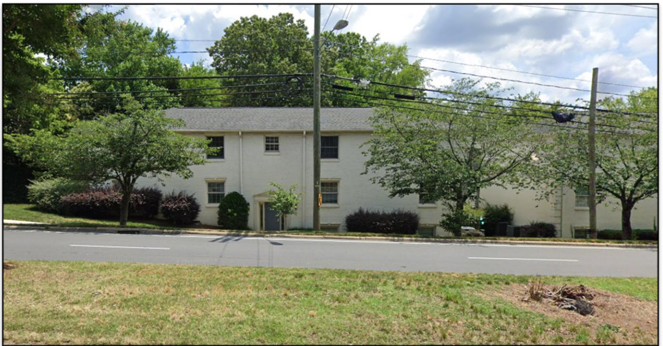
East of the site are multi-family dwellings.
