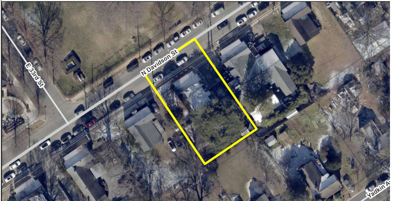
The site is surrounded by a mix of residential and nonresidential uses in the Noda community.
