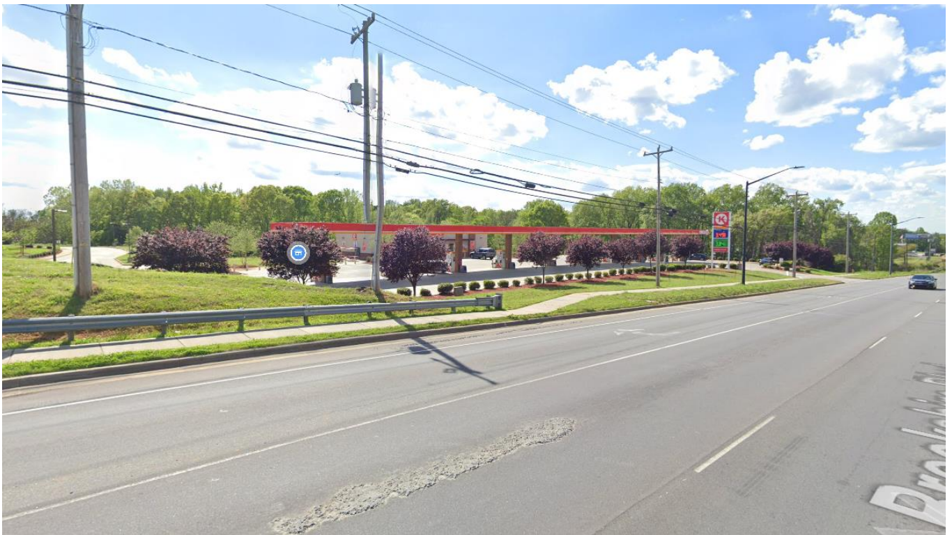
View of a gas station located to the north of the site across Fred D Alexander Blvd.
