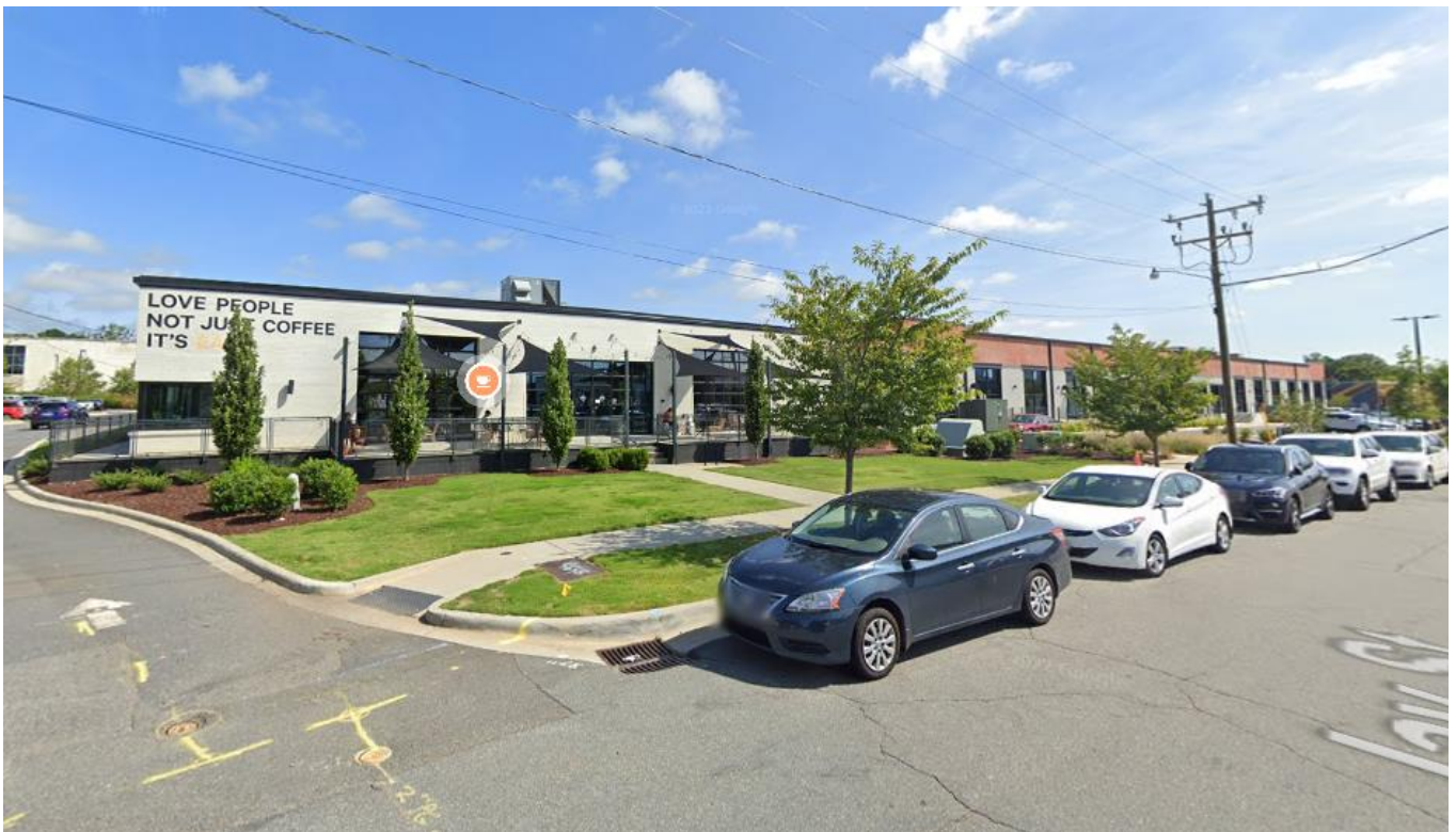
View of an adaptive reuse project along Jay Street, located southwest of the site, containing a coffee shop, office, and retail.
