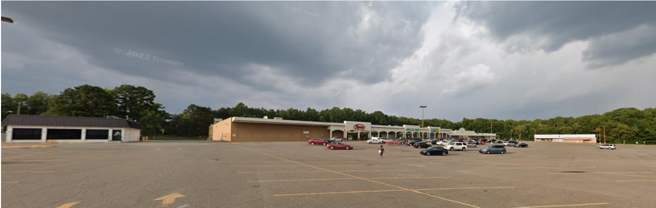
The subject site is developed with a shopping plaza and retail buildings.
