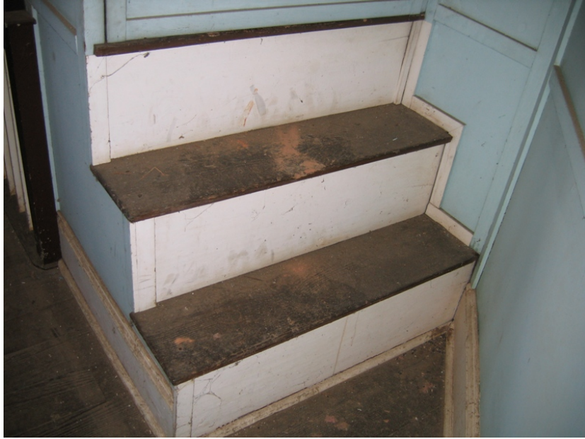
Steps leading to the enclosed attic stairway.
