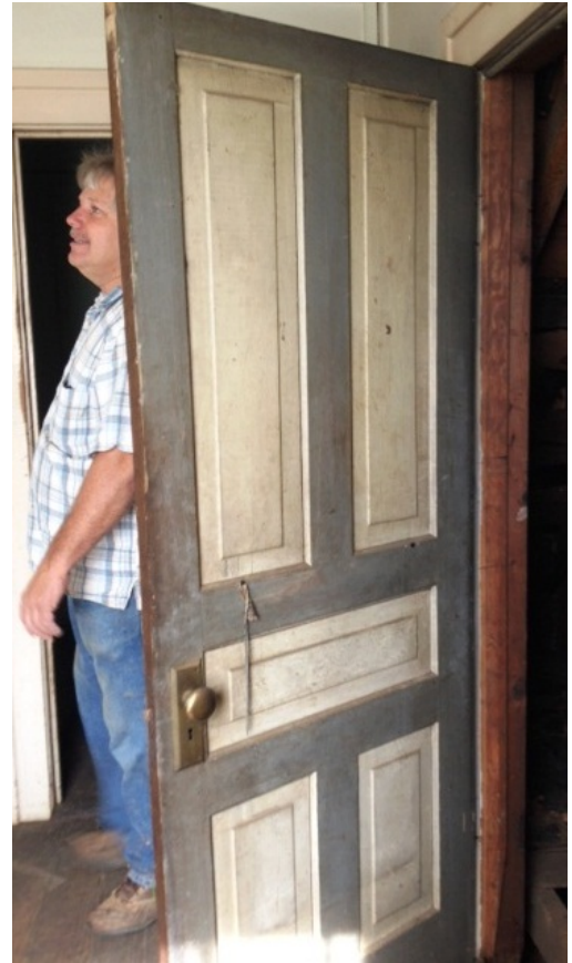
Late 19 th -century five-panel door.
