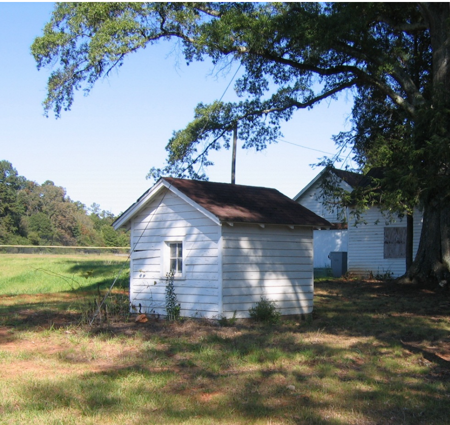
Located to the west of the house is a small well house built on a concrete slab. It features a narrow-board door with strap hinges, and exposed rafter ends. The rear elevation is pierced by a small, original, four-light window. The side walls are blank.
