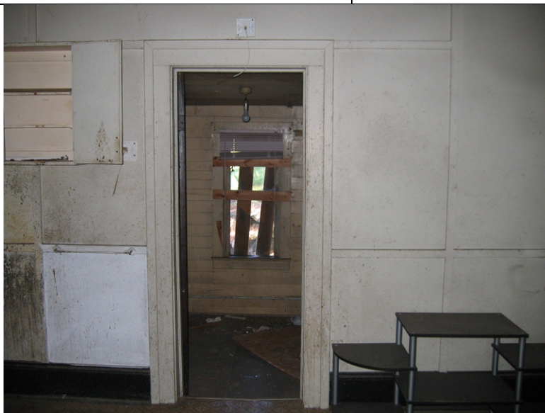
A view in the rear ell toward the rear of the house.
